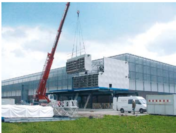
Placing Cooling Tower with crane on steel construction
